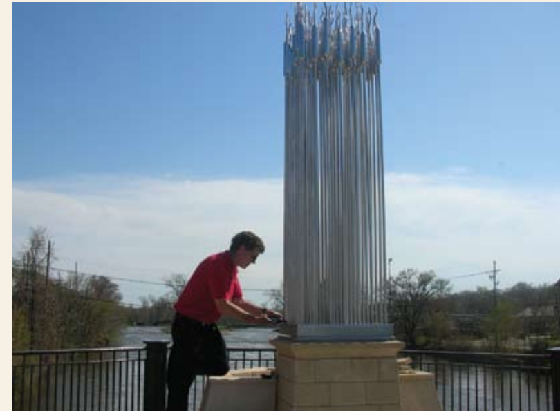
Kai Schulte's "Nature Sounds of Harmony" being installed on the Wilson Street Bridge.
