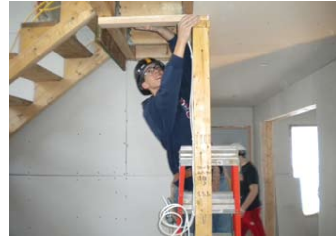
A student runs electrical wire for the house
