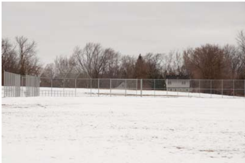
Below: The new diamond is completed. The fencing and the outline of the field is visible through the snow.
