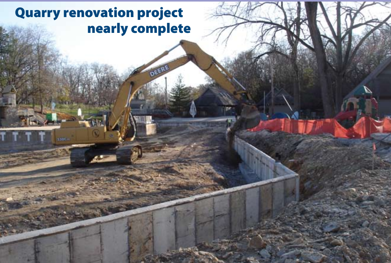
Backfilling the concrete wall.
